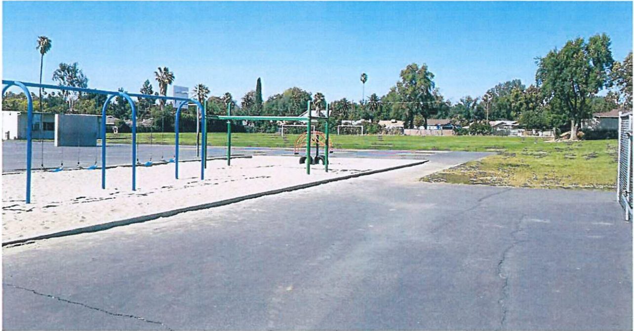
Photograph No. 1: Present site conditions in the area of classroom building
